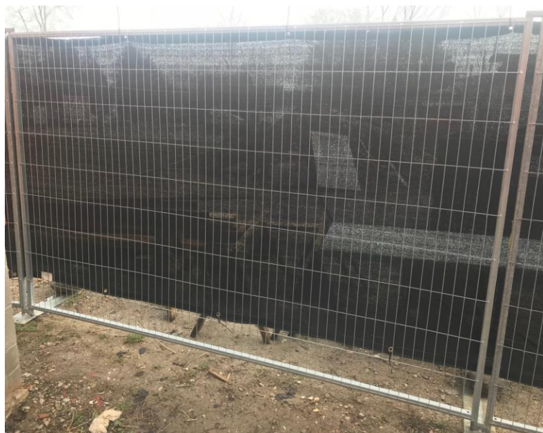
Image: Fence type to be used to protect public from access to construction area.
