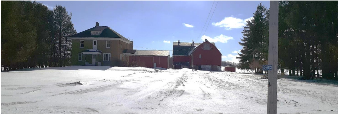
Figure 3.1: Site visit photo of severed surplus lot looking south from Belfast Road
