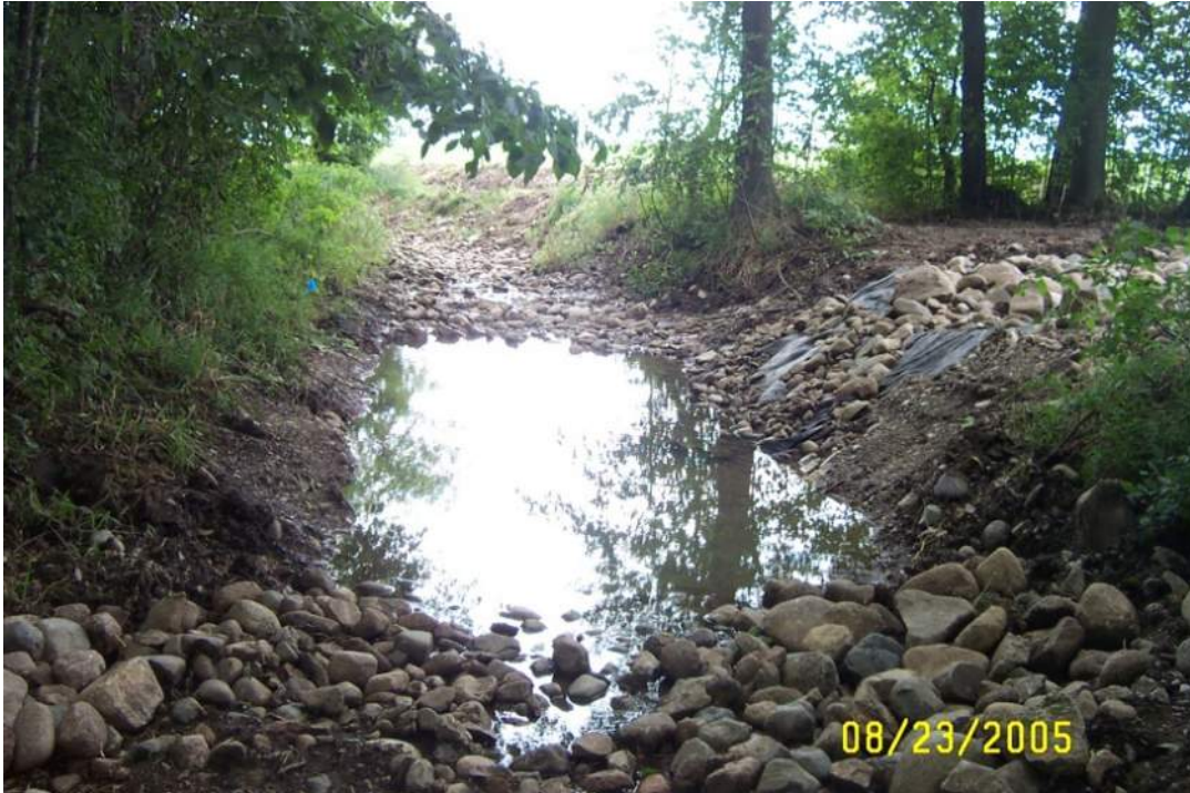
Figure 4 – Drain Pool and Spillway from Diversion Berm Overflow near Sta. 0+995
