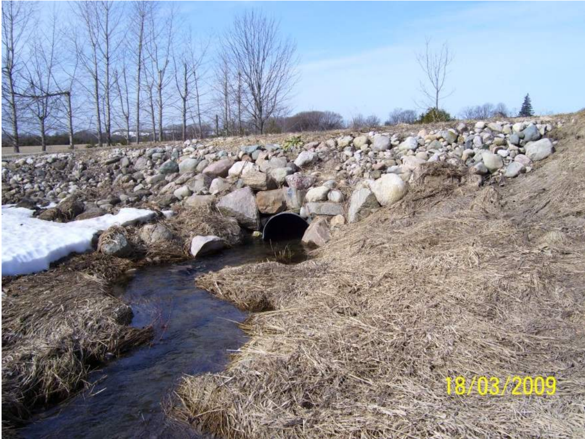
Figure 7 – Outlet of CSP Culvert Crossing on Scott Drain near Sta. 0+800
