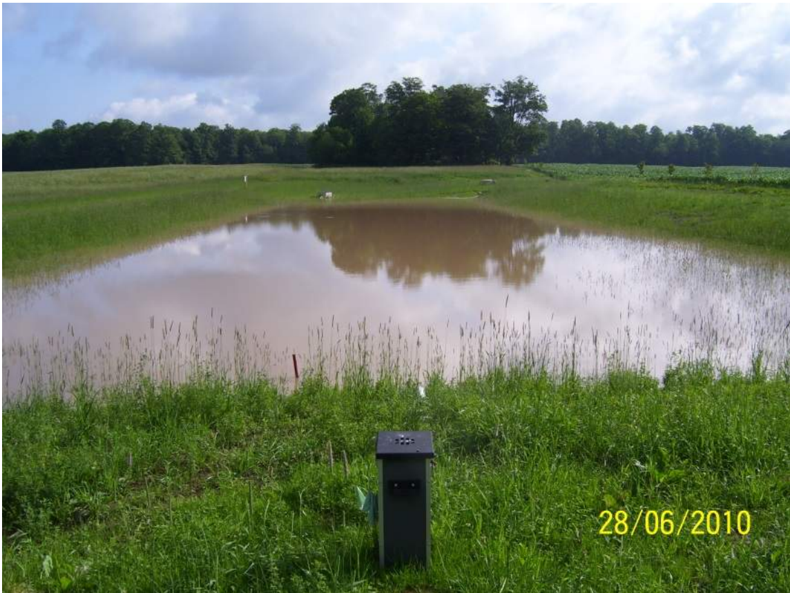
Figure 9 – Wetland A and Control Structure, Facing North
