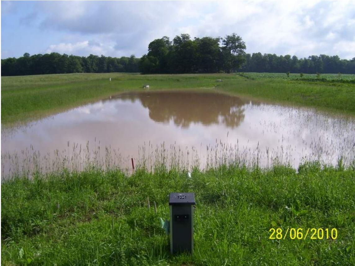
Figure 9 – Wetland A and Control Structure, Facing North
