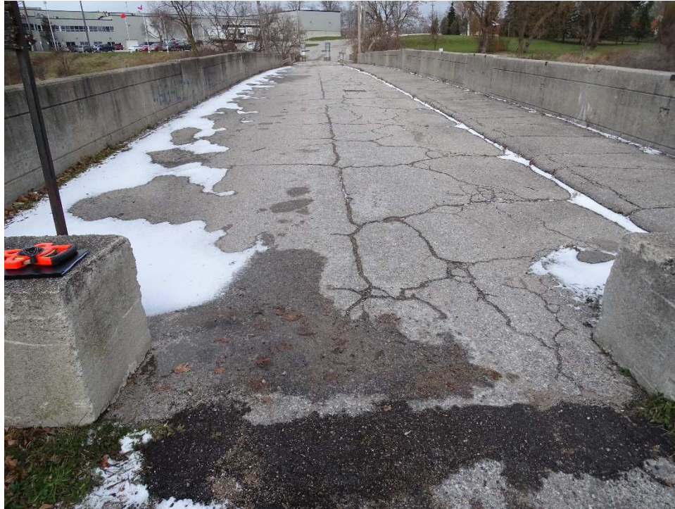
Photo 1 – Top of the Deck – Map Crack in Asphalt Looking North
