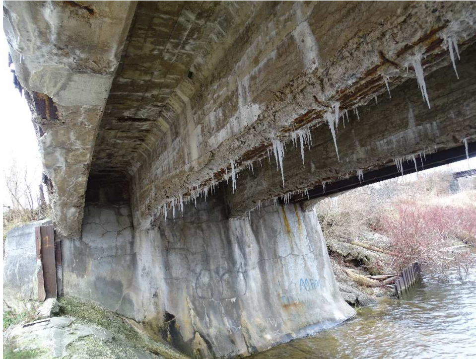
Photo 5 – Spalling and Exposed Corroded Rebar underside of the Girders and Deck – Span 4 Looking South
