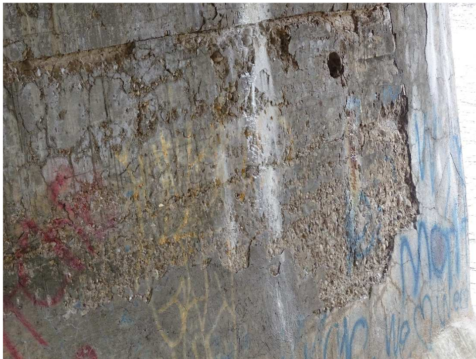
Photo 18 – Severe Spalling, Honeycombing and Hole in Pier 1 – Looking South
