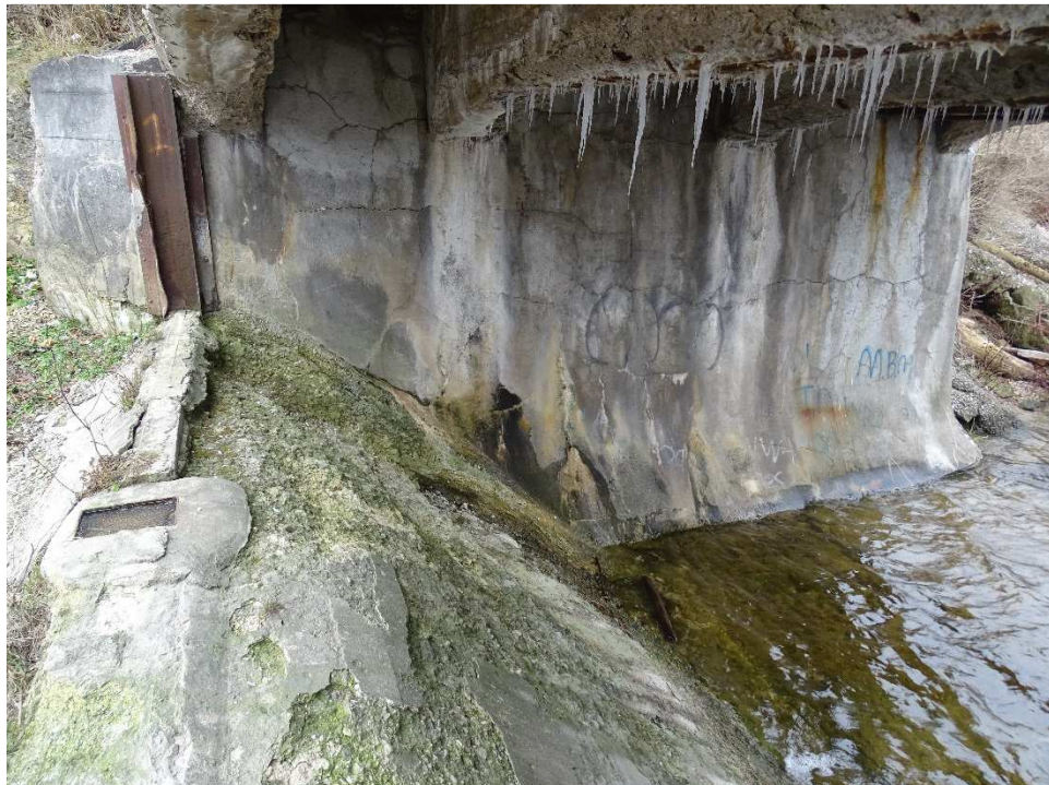
Photo 14 – South Abutment – Erosion, Joint Cold and Pattern Cracks
