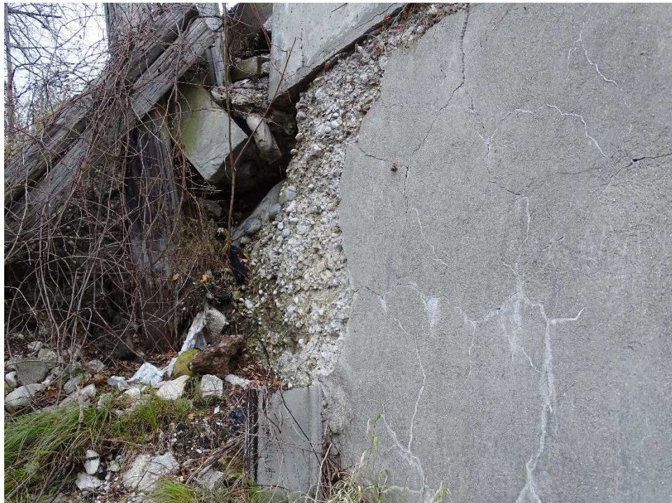
Photo 34 – North Downstream Retaining Wall - Spalling and Pattern Cracks
