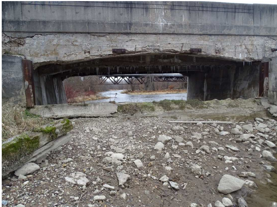
Photo 28 – Spalled Concrete – Upstream Weir of Span 4 (from North)
