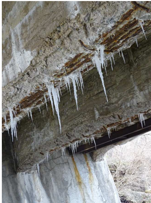
Photo 4 – Severe Spalled Concrete with Exposed Corroded Rebar underneath the Deck – Span 4
