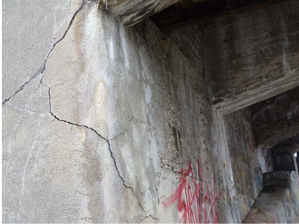
Photo 13 – North Abutment wide Crack - Looking Northeast
