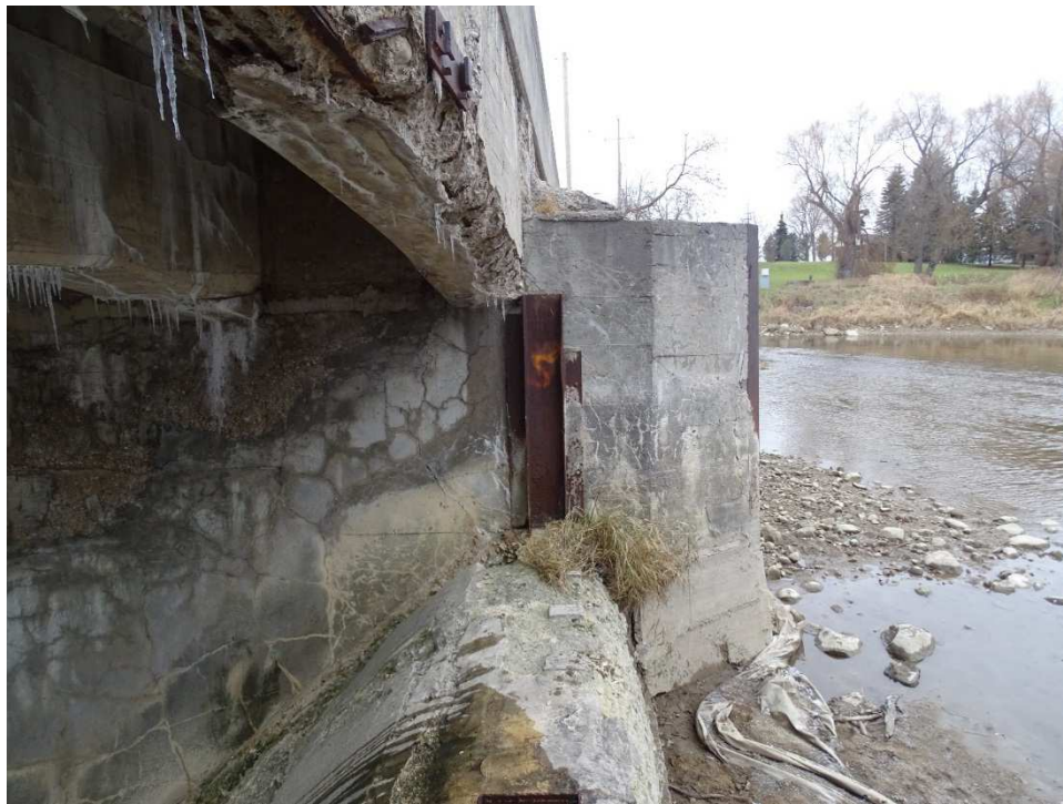
Photo 8 – Severe Spalling and Exposed Corroded rebar underneath the Girder – Span 3 Looking North
