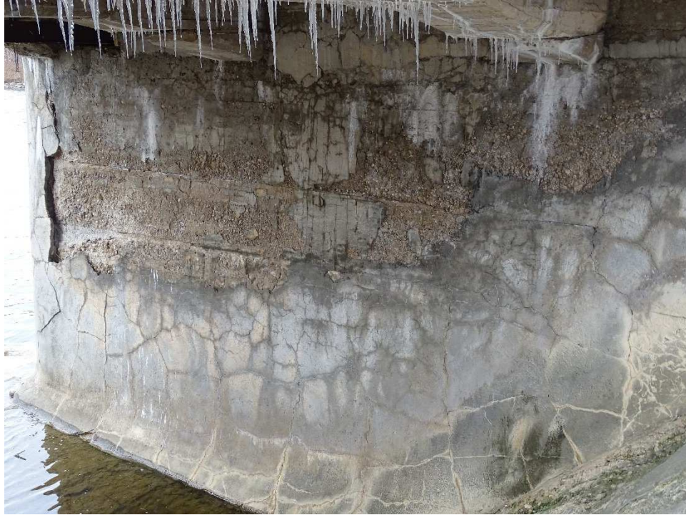
Photo 21 – Spalling on Pier 2 (from North) – Looking North
