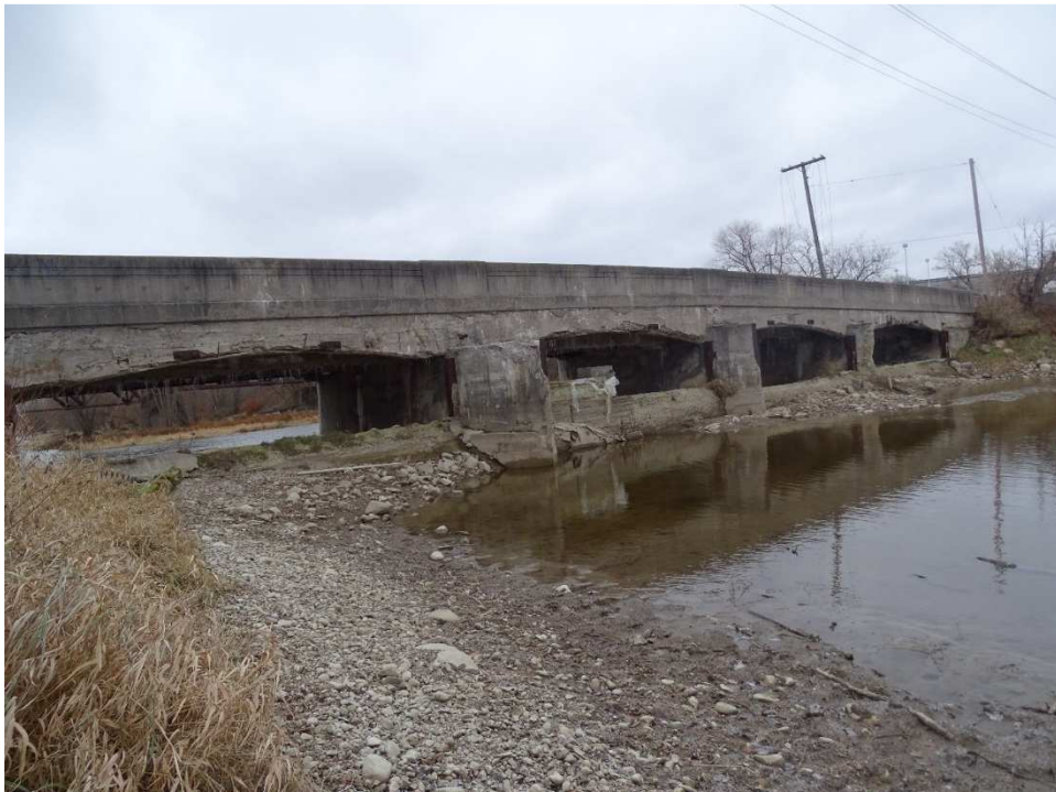
Photo 30 – Spalled Concrete – Upstream Weir Looking North
