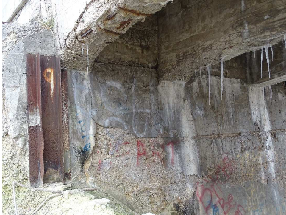
Photo 17 – Severe Spalling and Pattern Cracks on Pier 1 (from North) – Looking South
