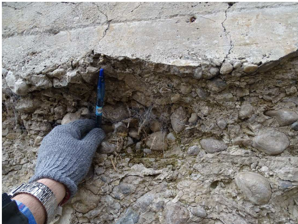
Photo 32 – North Upstream Retaining Wall – Severe Spalling
