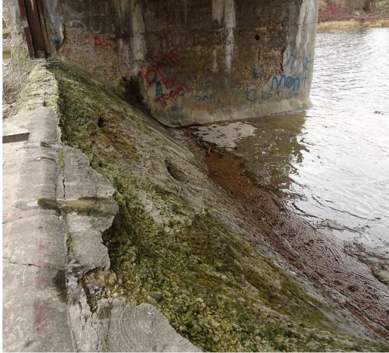
Photo 25 – Spalled Concrete – Downstream Weir of Span 1 Looking South
