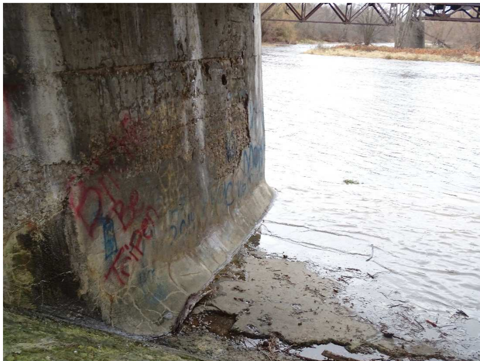
Photo 16 – Severe Spalling and Honeycombing on Pier 1 (from North) – Looking Southwest
