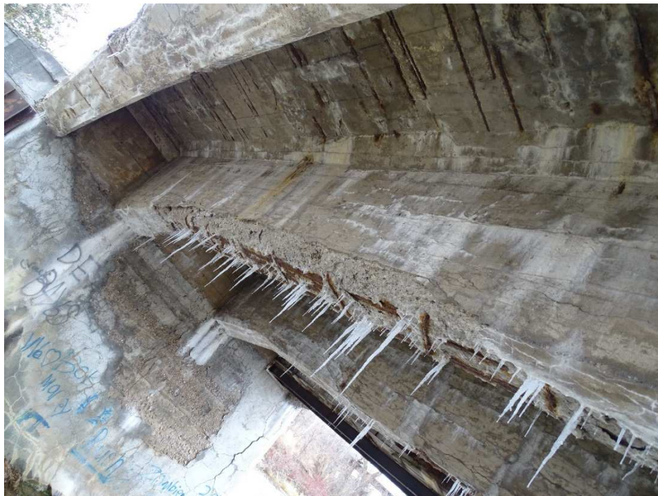
Photo 6 – Spalling and Exposed Corroded Rebar underside of the Girders and Deck – Span 2 Looking South
