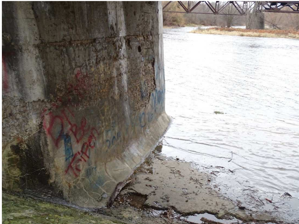
Photo 26 – Spalled Apron – Span 1 Looking Downstream
