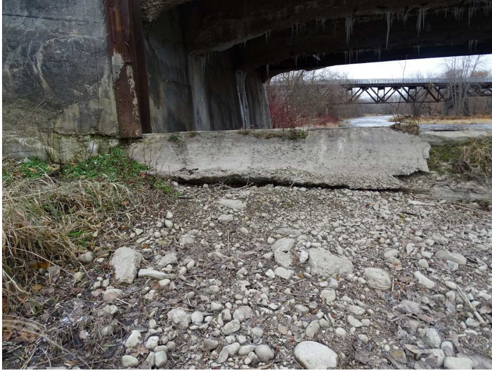
Photo 29 – Undercutting and Spalled Concrete – Span 4 (from North)
