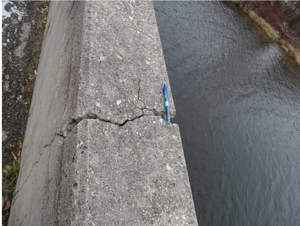
Photo 3 – Diagonal Crack in Parapet
