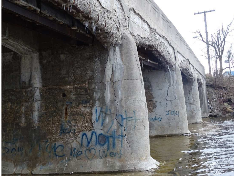
Photo 15 – Spalling and Pattern Cracks on Downstream of Piers - Looking South
