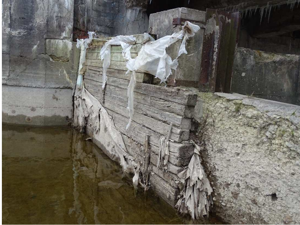
Photo 23 – Weathered and Decayed Stop logs – Looking South
