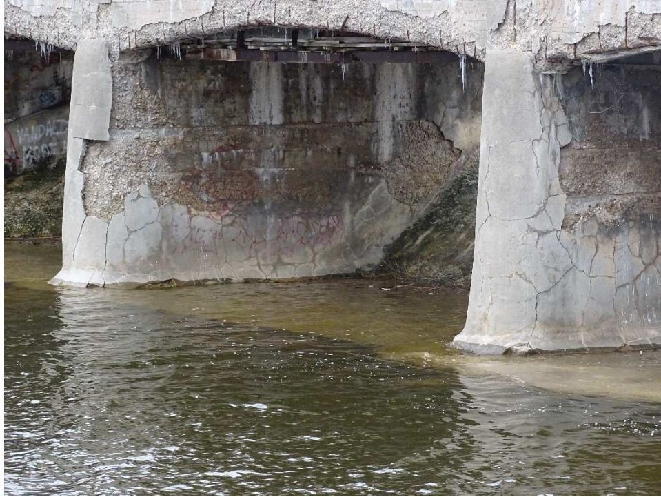
Photo 19 – Severe Spalling, Disintegration and Pattern Cracks on Pier 1 & 2 – Looking North
