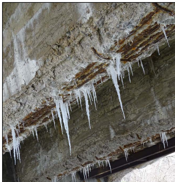
PHOTO 3.2.8 EXCESSIVE REBAR CORROSION AT GIRDERS
