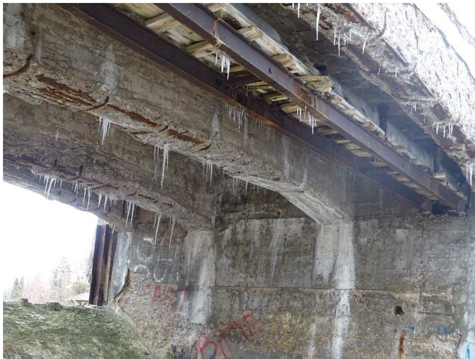
Photo 10 – Rusted Steel I Beam and Decayed Timber Transverse Beam– Span 1 Looking South
