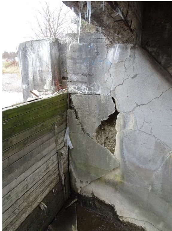
Photo 22 – Severe Disintegration, Spalling and Pattern Cracks on Pier 3 – Looking South
