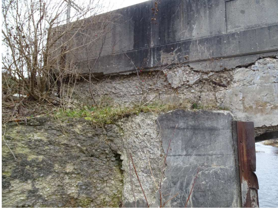
Photo 33 –South Upstream Retaining Wall – Severe Spalling
