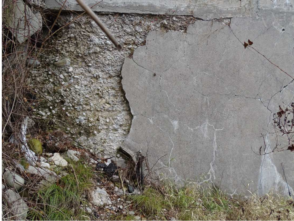
Photo 35 – North Downstream Retaining Wall - Spalling and Pattern Cracks
