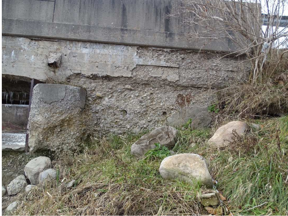
Photo 31 – North Upstream Retaining Wall – Severe Spalling
