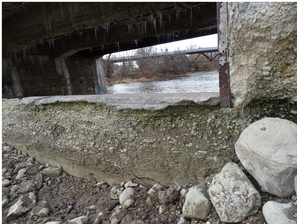
Photo 24 – Spalled Concrete – Upstream Weir of Span 1 (from North)
