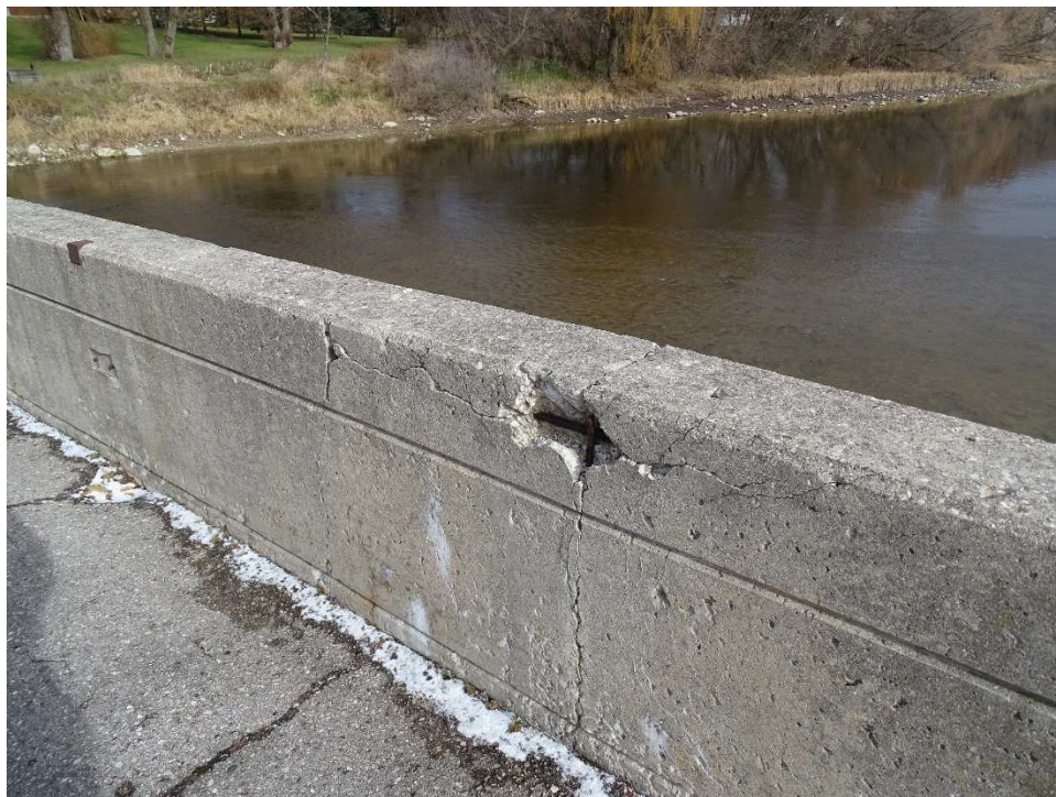
Photo 2 – Spalled Concrete and Exposed Rebar in Parapet - Looking Upstream
