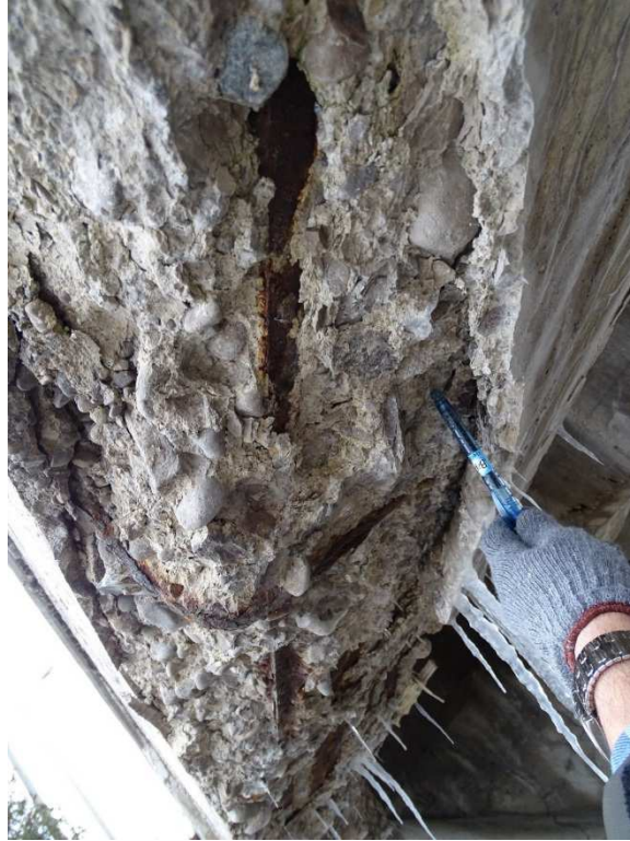
Photo 7 – Icicles underneath the Girders with Severe Spalling and Exposed Corroded Rebar – Span 3
