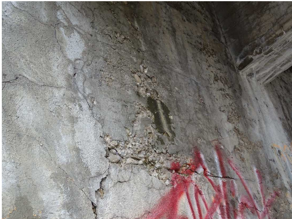
Photo 12 – North Abutment Spalling and Honeycombing – Looking North
