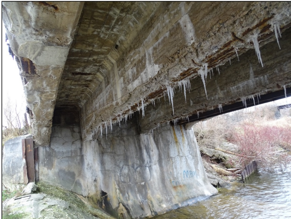
PHOTO 3.2.8 EXCESSIVE REBAR CORROSION AT GIRDERS
