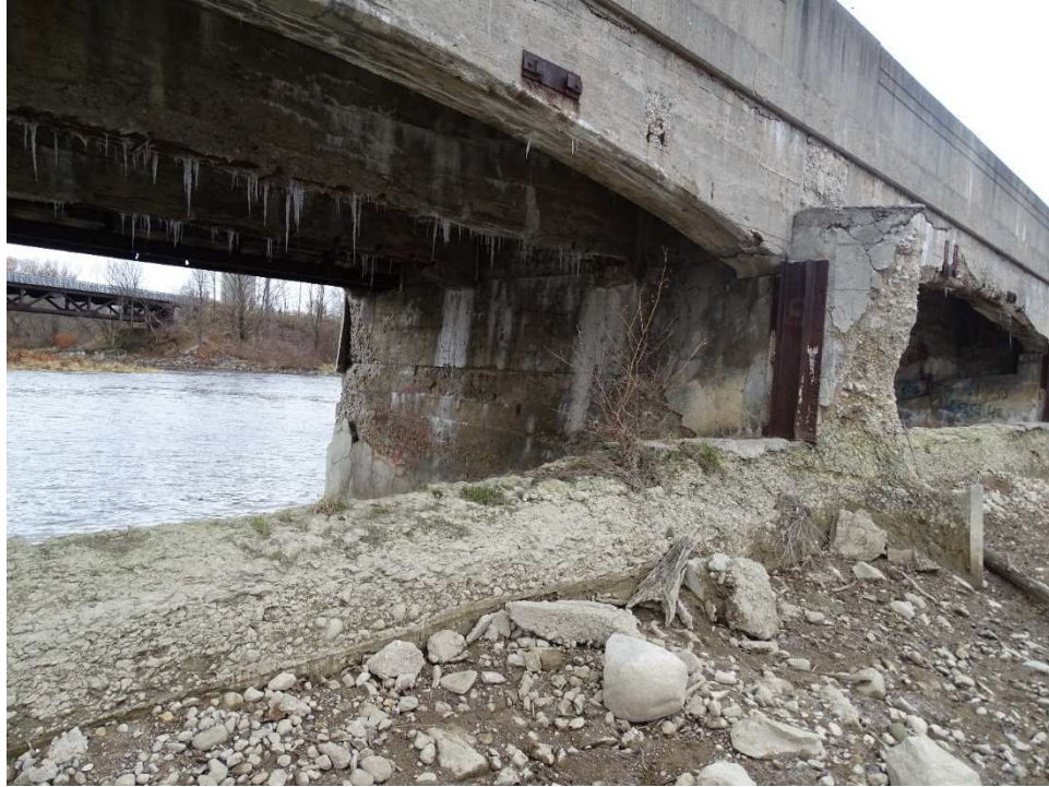
Photo 27 – Spalled Concrete – Upstream Weir of Spans 1 & 2 (from North) Looking North
