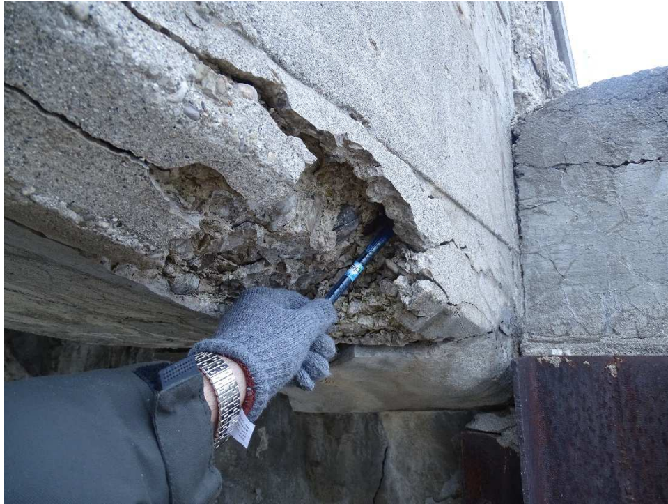
Photo 9 – Severe Spalling underneath the Girder – Span 2 Upstream
